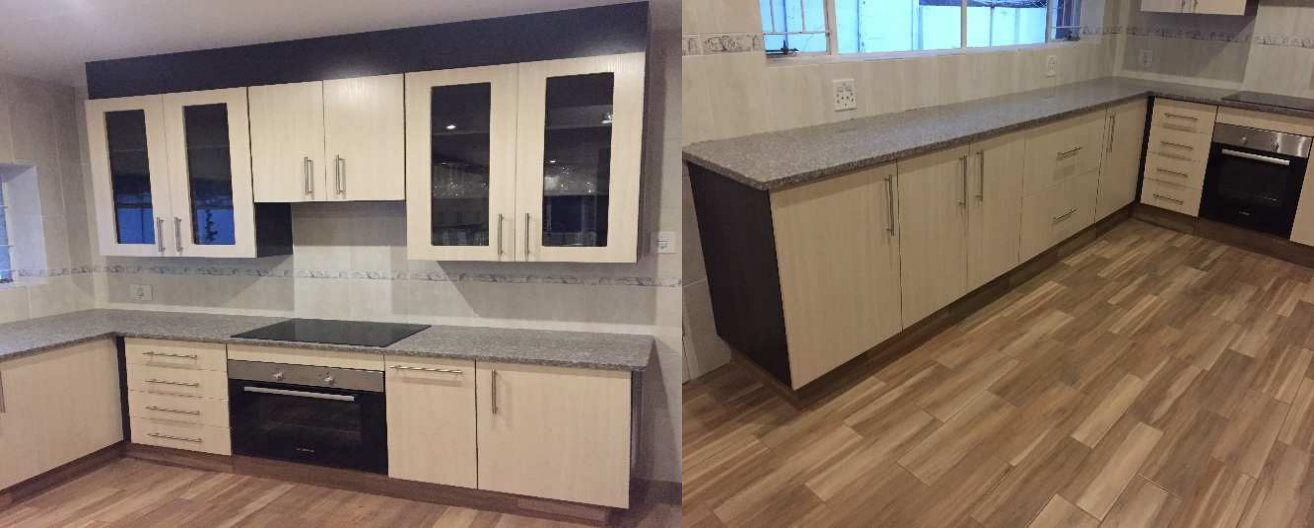
Actual Kitchen after Installation Cost Of Kitchen R 91,977.00 Excluding Granite, Appliances and Installation
